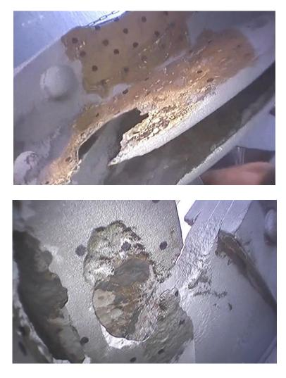
*Photo source: video by Faculty of Civil Engineering, CTU, corrosion captured by endoscopic probe on the diagonals of the Výtoň bridge, September 2023*
