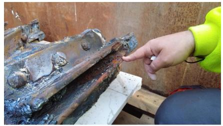
Photo source: video by Správa železnic, testing by Faculty of Civil Engineering, CTU – corrosion in the place of the vertical of the Děčín bridge
